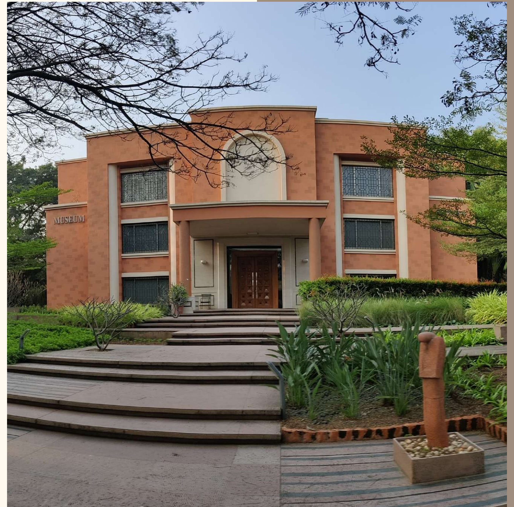
Museum Building, Vidya Pratishthan, Baramati
