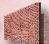
LATERITE BRICK WALL
